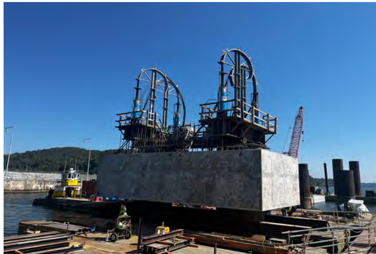
Upstream intermediate pier after first placement
