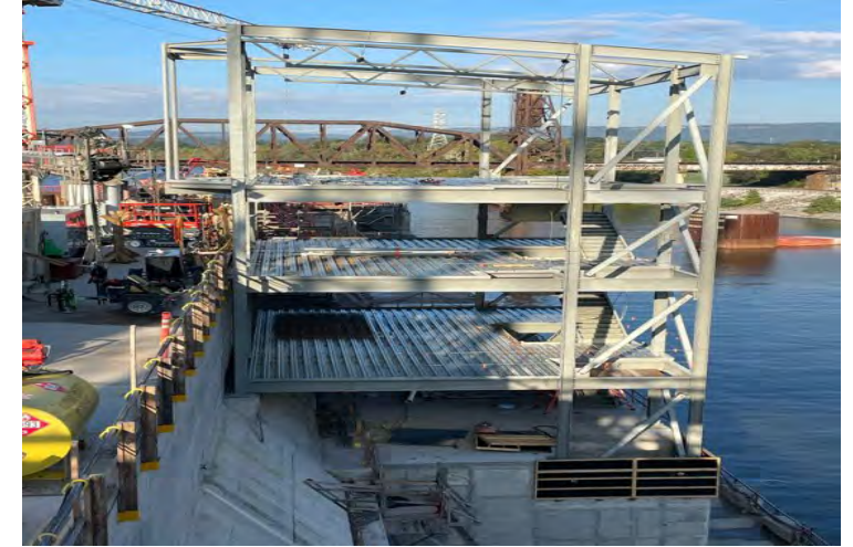
Operations Building, Steel Framing near completion.
