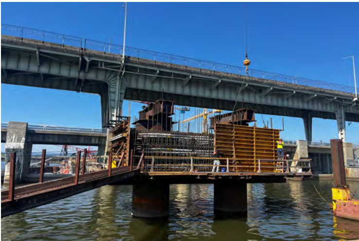
Upstream intermediate pier formwork
